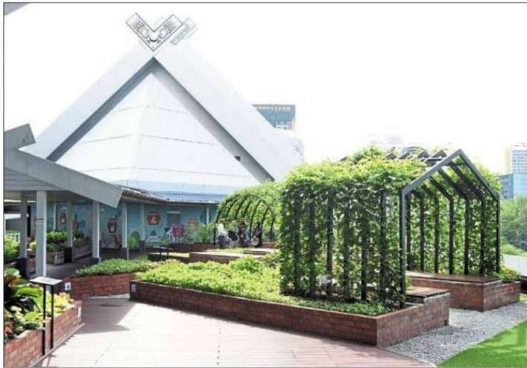
The Wisma MBSA rooftop now has an edible garden that also offers a cool respite for employees. — KK SHAM/The Star
