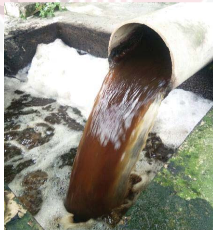
Figure 1.1: Final discharge of POME in Maran, Pahang
