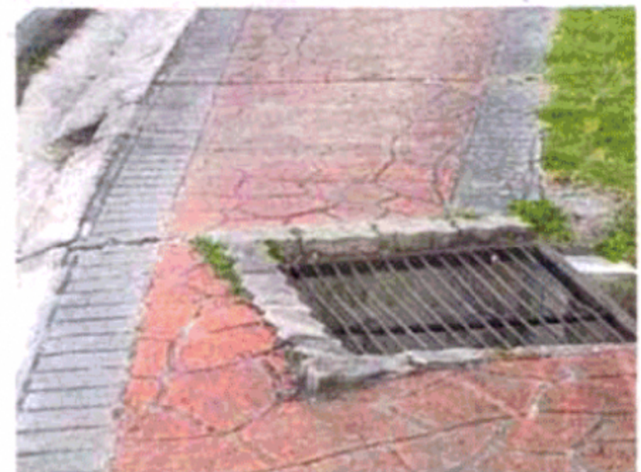
Example of a roadside pathway that is 'interrupted' by a drain cover.
