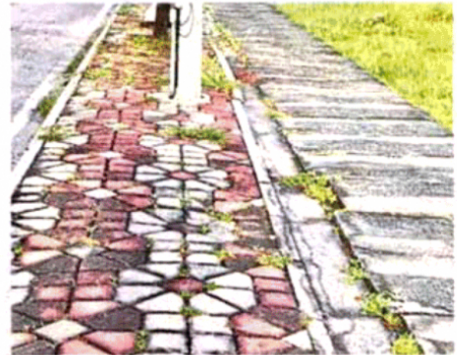
Unsuitable material for a walkway, made worse with a lamp post in the centre.
