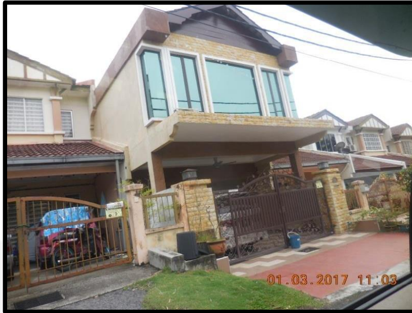
Figure 1.1: Extension of the Porch Blocking Natural Light and Ventilation
