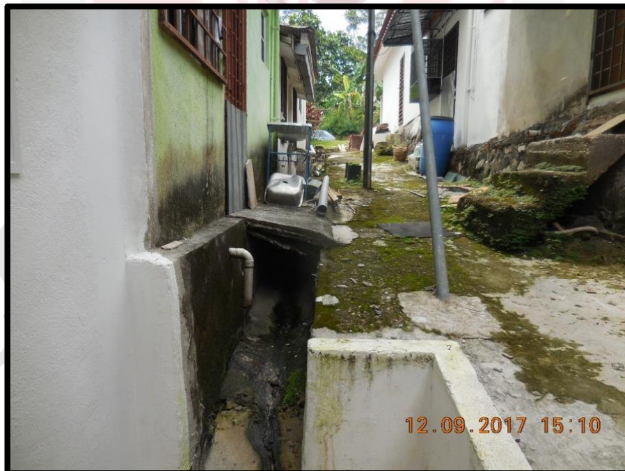
Figure1.2: Wastewater Channelled Directly into the Perimeter Drain
