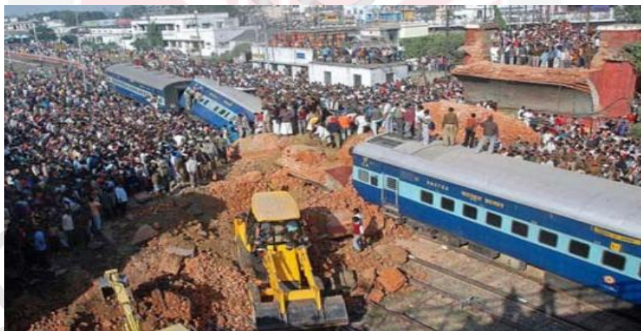
Figure 1.3 : Collapse of Railway Bridge near Bhagalpur (Shanker, 2009)
