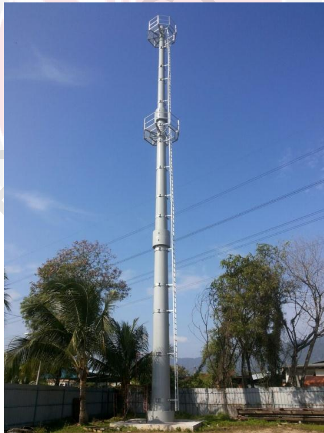
Figure 1.5 : Communication tower with 30 m height located in Malaysia
