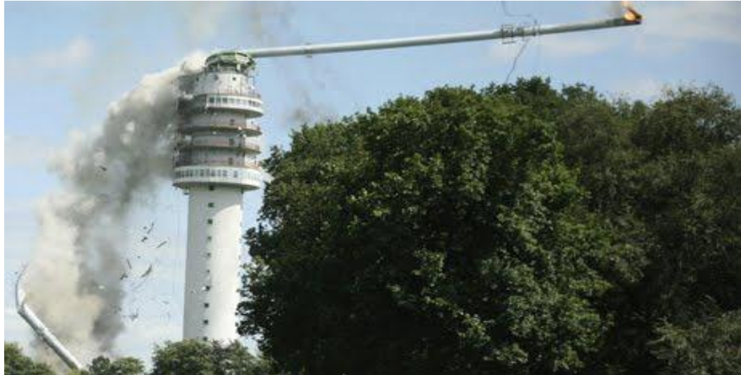
Figure 1.4 : Collapse of 300m communication tower mast in northern Netherlands
