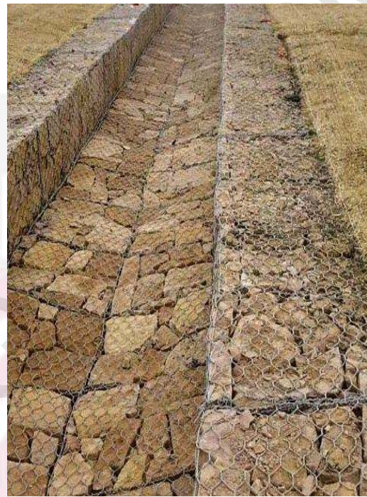
b) Gabions channel
