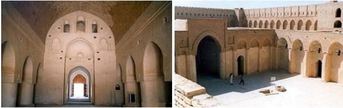
Figure 1. Pointed barrel vault and arches of the great hall of Al-Ukhaidhir Palace – Source: https://www.cemml.colostate.edu Figure 2. The Northern side of the court of honor and the upper floor of Al-Ukhaidhir Palace – Source: https://www.cemml.colostate.edu
