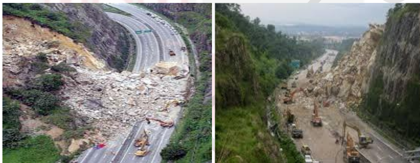
Figure 1.1 Rockfall Incidents along the North-South Expressway
