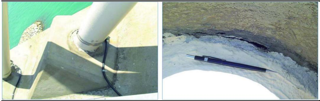
**Figure 1.2 : Structural defect of cable Anchorage with bridge girder**
