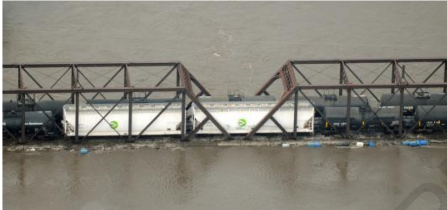
Figure 1.1. Flood waters submerge bridge and surround freight cars in Iowa in 2008 (Associated Press, 2008).
