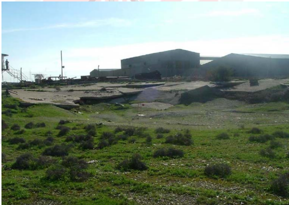
Figure 1.3 : Sinkhole Below Concrete Paved Area (SIGIR, 2007)
