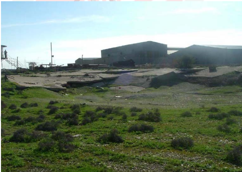
Figure 1.3 : Sinkhole Below Concrete Paved Area (SIGIR, 2007)
