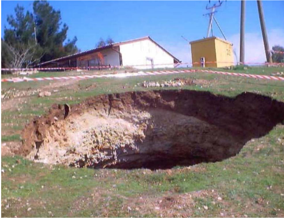
Figure 1.2 : Sinkhole About 500 m Downstream from the Dam (SIGIR, 2007)
