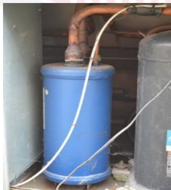
Figure 1.2: Air conditioner hot gas receiver tank
