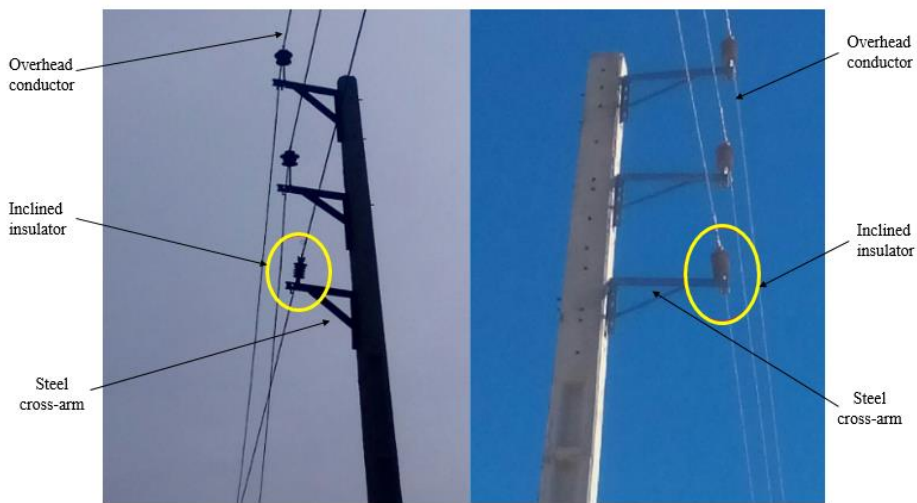
Figure 1.1: The inclination of insulator during the operation
