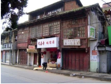
Figure 1.1 – Old utilitarian shophouses in Kunming, China. Image Source: http://www.greatmirror.com
