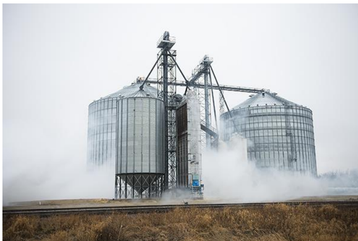
Figure 1.1: Leakage in an anhydrous ammonia tank in Clarks Grove [5]
