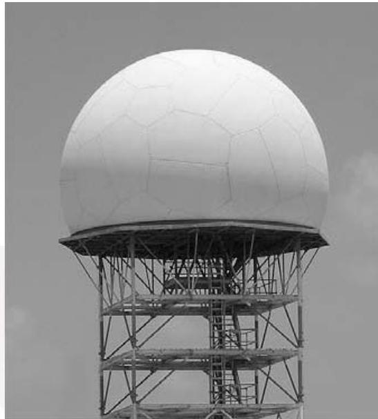
**Figure 1.4: Radome-enclosed air traffic control radar antenna. [11]**
