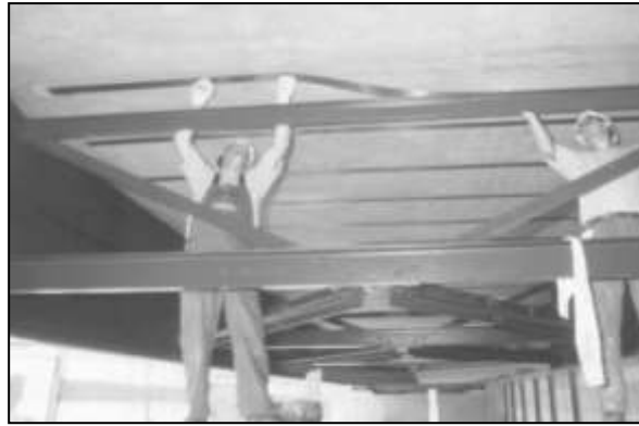
Figure 1.4 : EB Method of FRP plate (Thanasis et al. , 2001)
