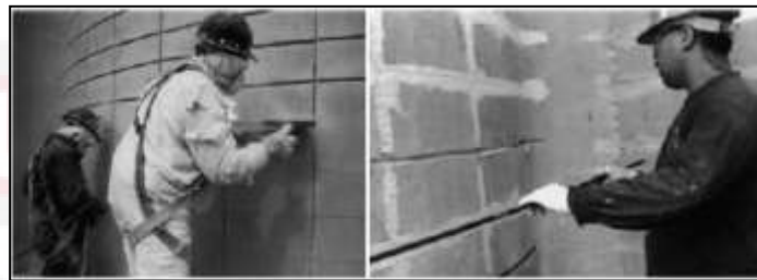
Figure 1.5 : NSM method of FRP plate (Alkhrdaji and Thomas, 2006).
