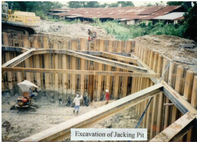
Plate 1: Construction of the jacking pit Source: DID, Negeri Sembilan
