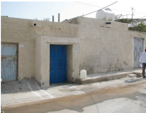
Fig. 20: A typical entrance, Old Saffein
