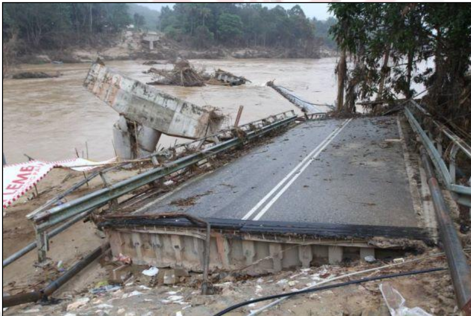
Fig.1.4: Stelu River Bridge at Gua Musang, Kelantan, collapsed due to scouring during floods
