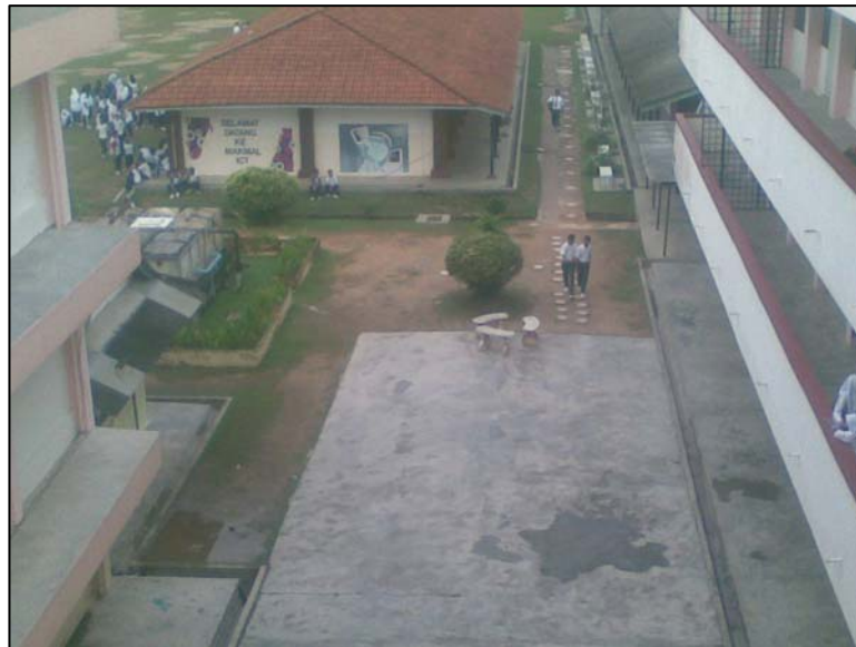
Figure 1.1: The cement pavement in school compound
