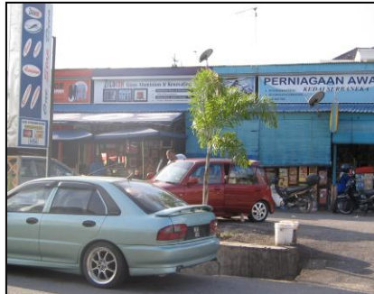
Single storey shophouses/shopoffices
