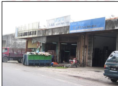
Single storey industrial terraces
