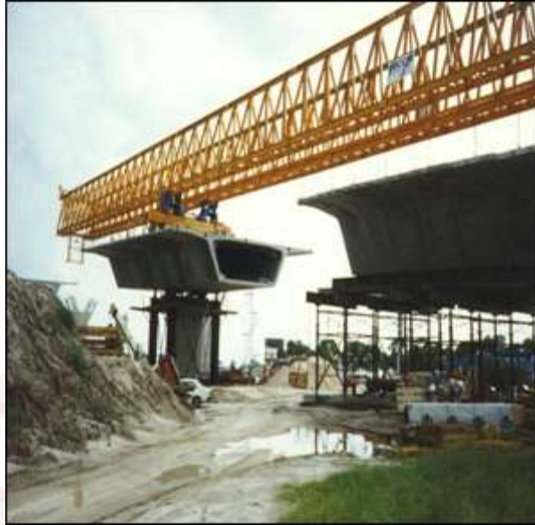
Fig.1.1: Second Link Bridge to Singapore during construction
