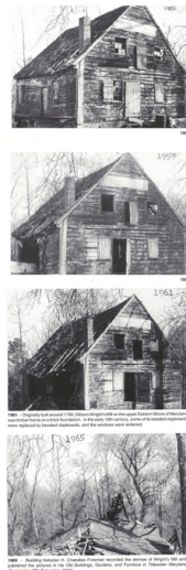
Figure 3 : WHO BUILDS IN WOOD build a shack – adaptable now, gone soon. No other material is so easy to work, and none is so vulnerable to neglect, except maybe adobe. Once roof and windows of Wright's Mill were open, even its sturdy timber frame construction could not save it from the effects of constant moisture. To insects and fungus, wet wood is food.
