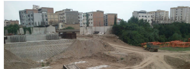
Figure 4: current condition of residential area around the Riverside.
