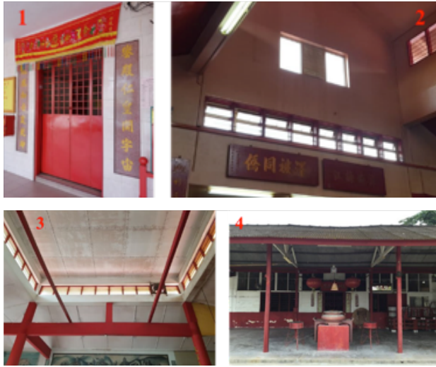
Figure 3: Design character- without the classical design identity and replace with modern materials. Image 1&2: Xian Shi Temple in Semenyih, Image 3: Nam Tian Gong in Ulu Yam, Image 4: Xian Shi Temple in Sungai Tekali. Source* Author 2018
