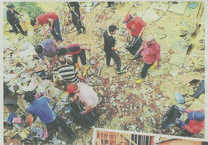
What a mess: Universiti Putra Malaysia volunteers worked hard to clear the destroyed items from the thick layer of mud in Rantau Panjang and Pasir Mas, Kelantan. As many as 150 volunteers from the varsity were involved in the effort.
