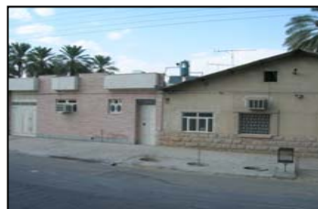
Figure 7: The sloped roof illustrates the form of original post-earthquake housing and seemed uncoordinated with the flat rooftop of the new extension to suit the local condition (source: Muhammad Parva, 2009)
