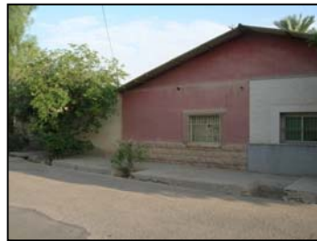
Figure 6: A Post-Earthquake House façade (semi-detached houses sharing sloped roof and a wall). (Source: Muhammad Parva, 2009)
