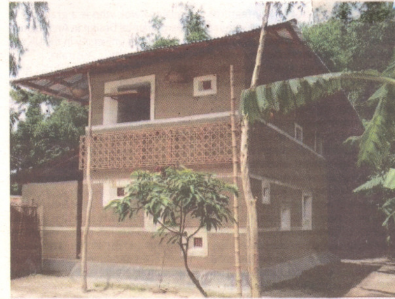
A house made of mud and bamboo in the rural area of Rudropur, Bangladesh.
