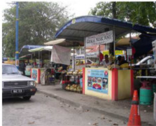
Figure 4: Current problems in microarchitecture in Malaysia: Designed street micro stall made from unsuitable materials.
