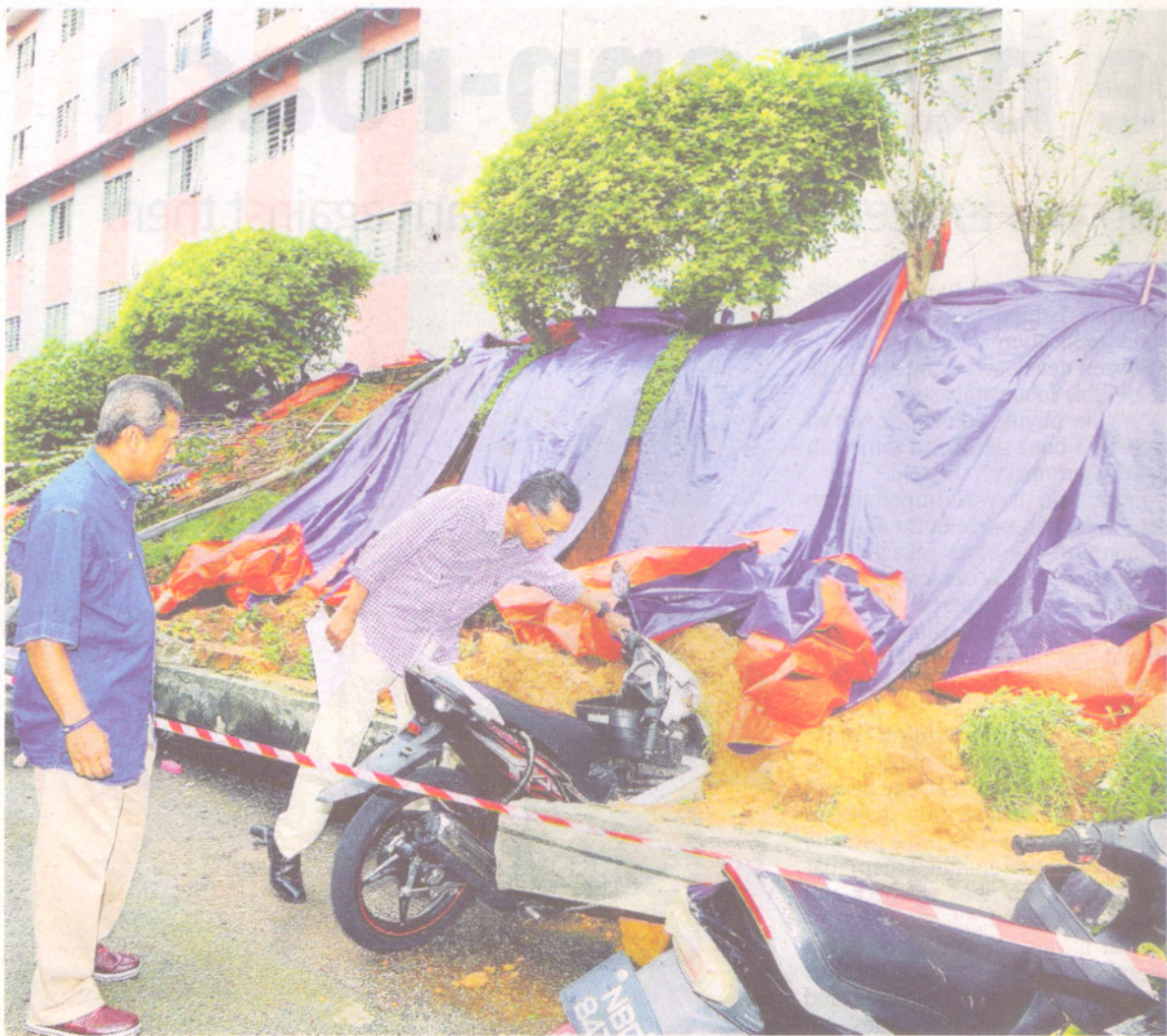
Can't let it slide: Shaziman (right) inspecting the landslide site at UPM in Serdang. — Bernama
