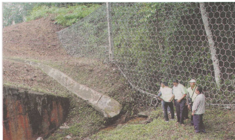
SECURITY: One of the five debris flow nets installed at Gua Tempurung and Jelapang.
