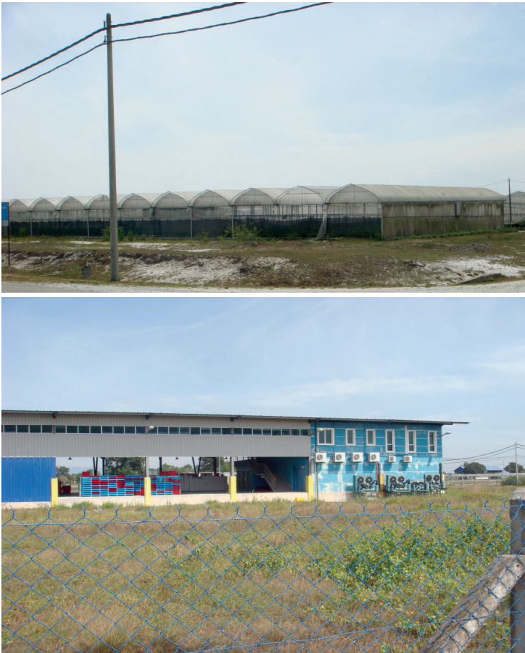
Figure 3 One of the state government agricultural agencies ventures with expertise from Holland involving an investment of approximately RM 4 million. The project was initiated in 2006 and at present was abandoned and failed to meet the objective of increasing food production and to improve farmers' income.
