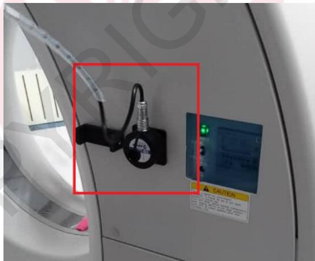
Figure 4.3: MK926 MEMS accelerometer attach on gantry to detect the vibration of the machine.
