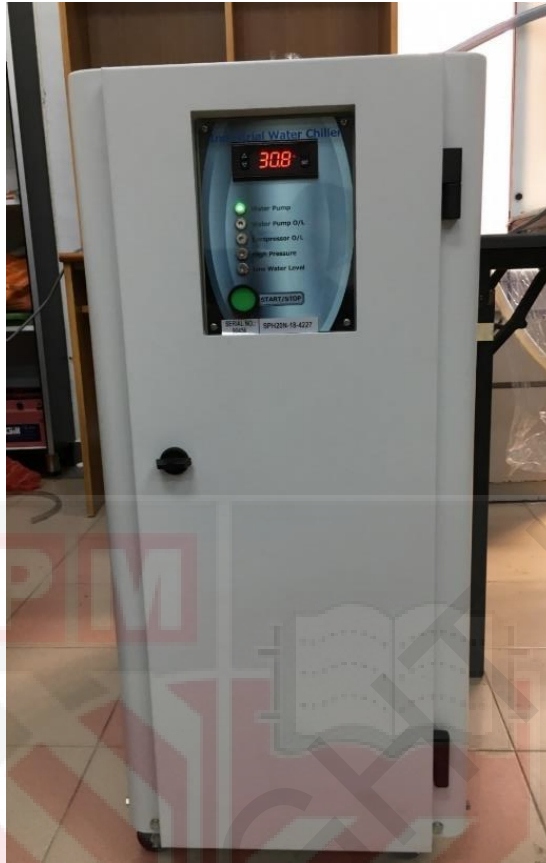
Appendix B4. Industrial water chiller
