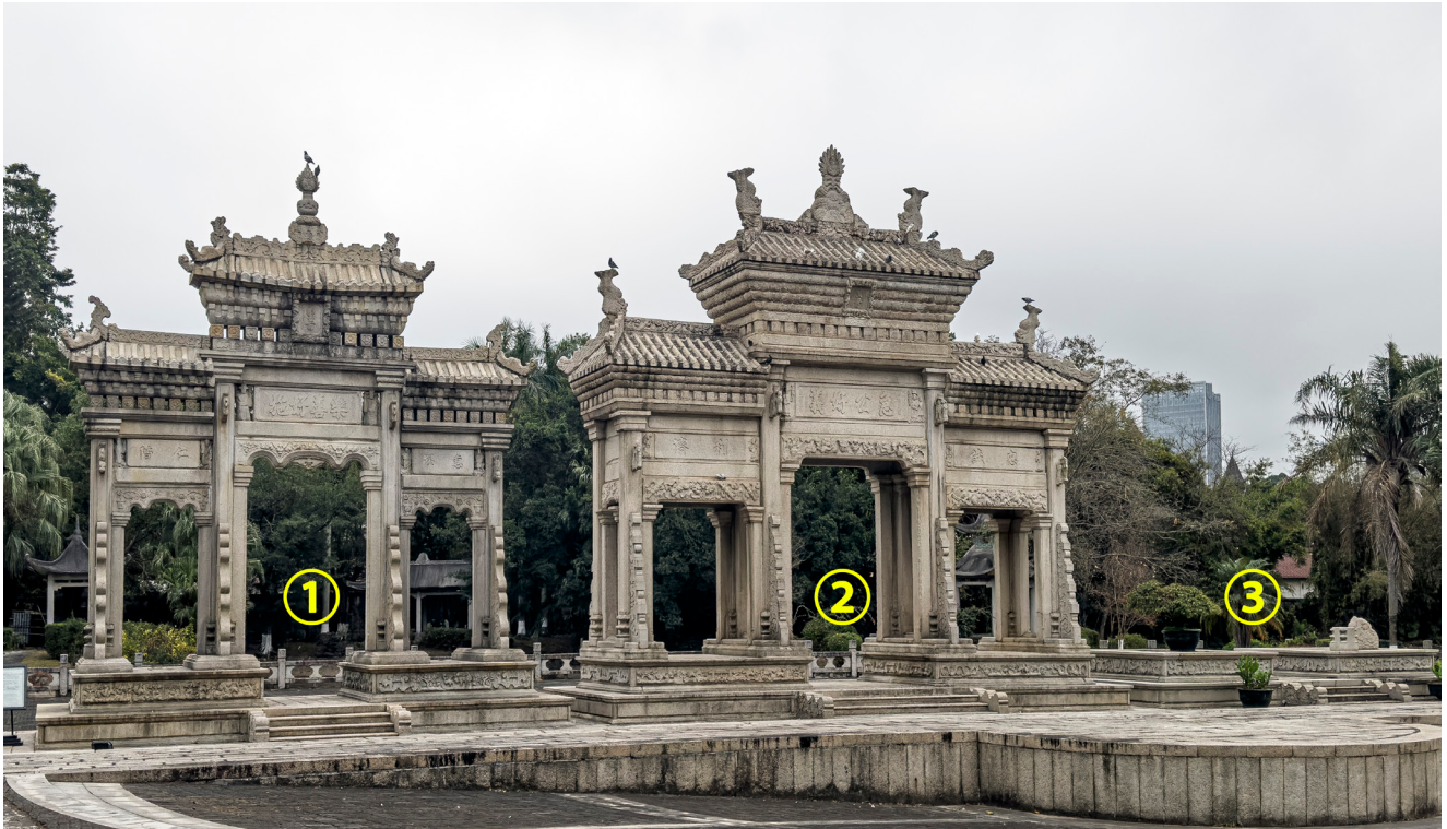
Figure 4: View towards ①-③.
