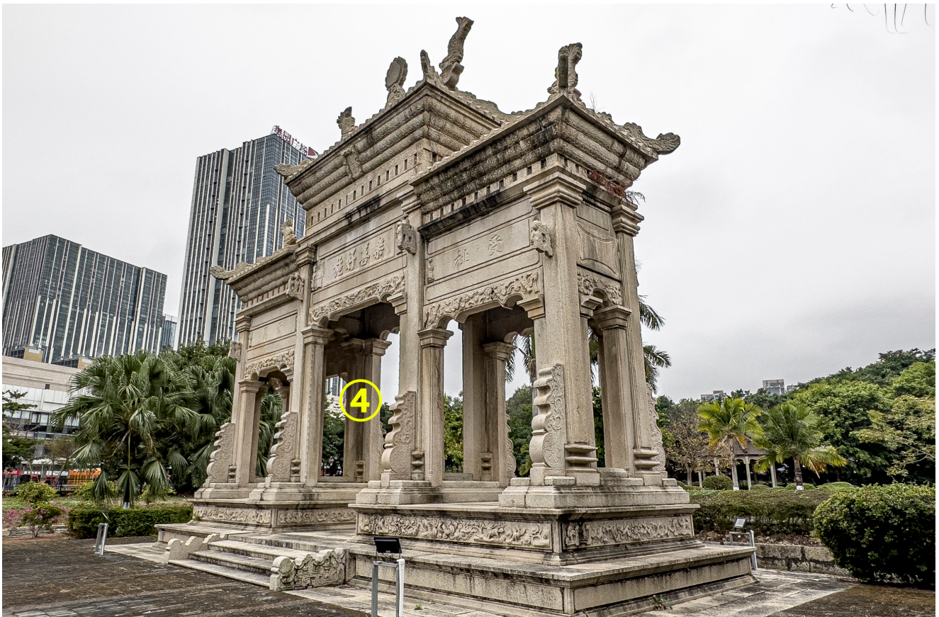
Figure 5: View towards ④.
