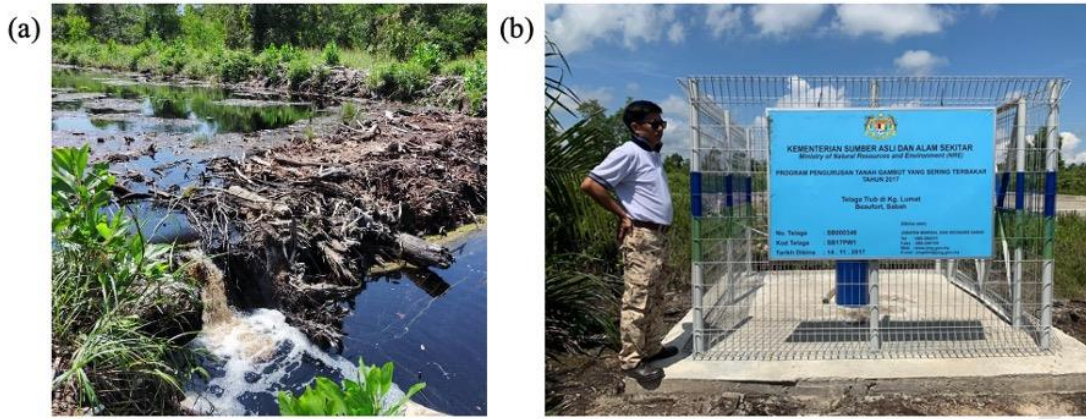
Figure 6: (a) Canal implemented in Klias Forest Reserve as a fire break to prevent fire spread from state land and plantation nearby; (b) District Forest Officer of Beaufort, standing beside the tube well in Kg. Lumat, Beaufort, and Sabah to help in fire suppression. (Source: Dayang Nur Sakinah Musa)
