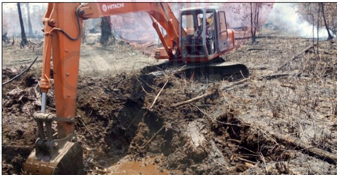
Figure 44: Construction of a pond for water supply during the prolonged drought in addition to El-Niño, which was present in 2016 affected most areas of Sabah including the Binsuluk Forest Reserve. (Source: Sabah Forestry Department).
