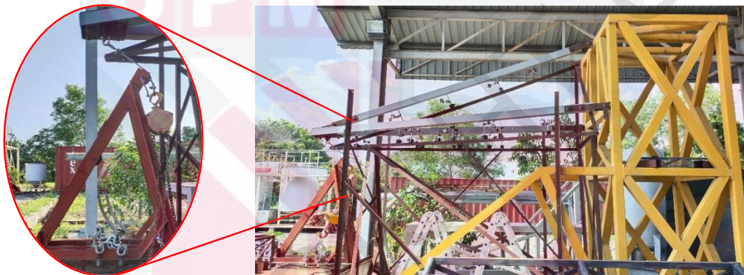
Figure 3.19: Actual PGFRPC cross-arm condition during normal wire condition test.
