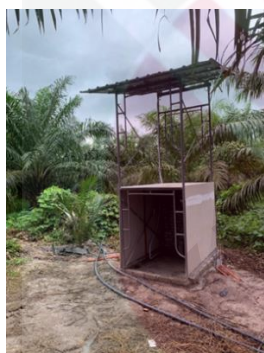
Figure D.11: A photovoltaic panel was installed at the roof of this structure
