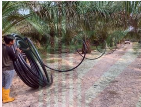
Figure 3.29: The coiled HDPE was stretched along the main road
