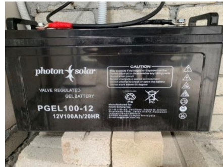
Figure D.14: Deep cycle battery used to store to energy
