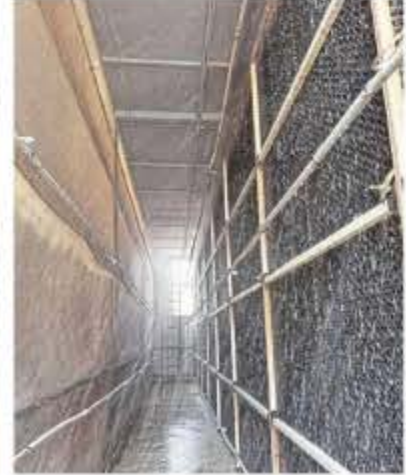
Odour-control at QL Poultry Farms involves a system with mist and deodoriser.
