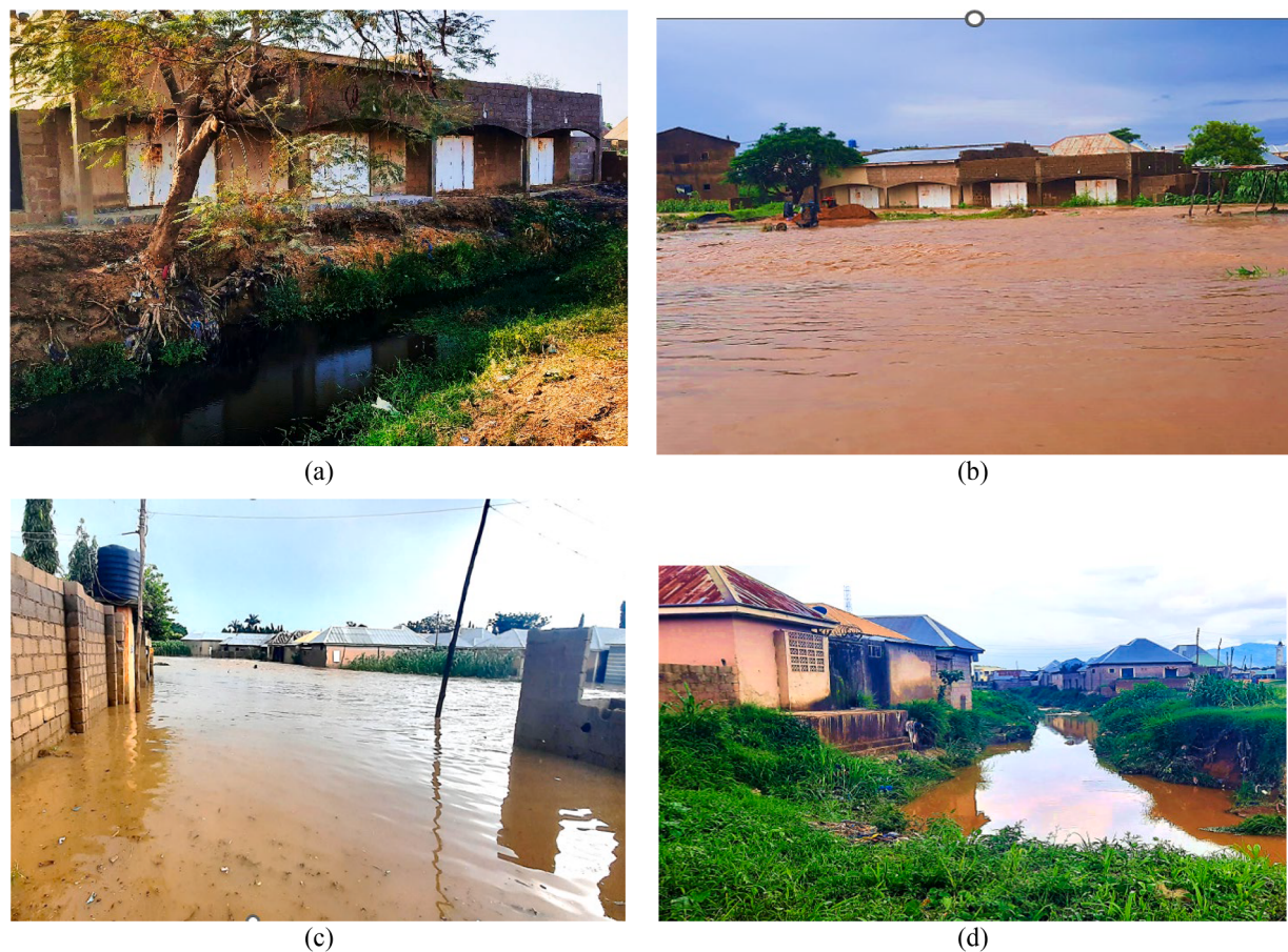
Fig. 6. Flood incidences (a) commercial development encroaching on a water way along Federal Low-cost Bye-pass, (b) the same commercial building submerged by the 4th September 2024 flooding, (c) Bayan Kotu completely submerged by the 4th September 2024 flooding and (d) Bayan kotu showing arrangement of buildings along water channel.
