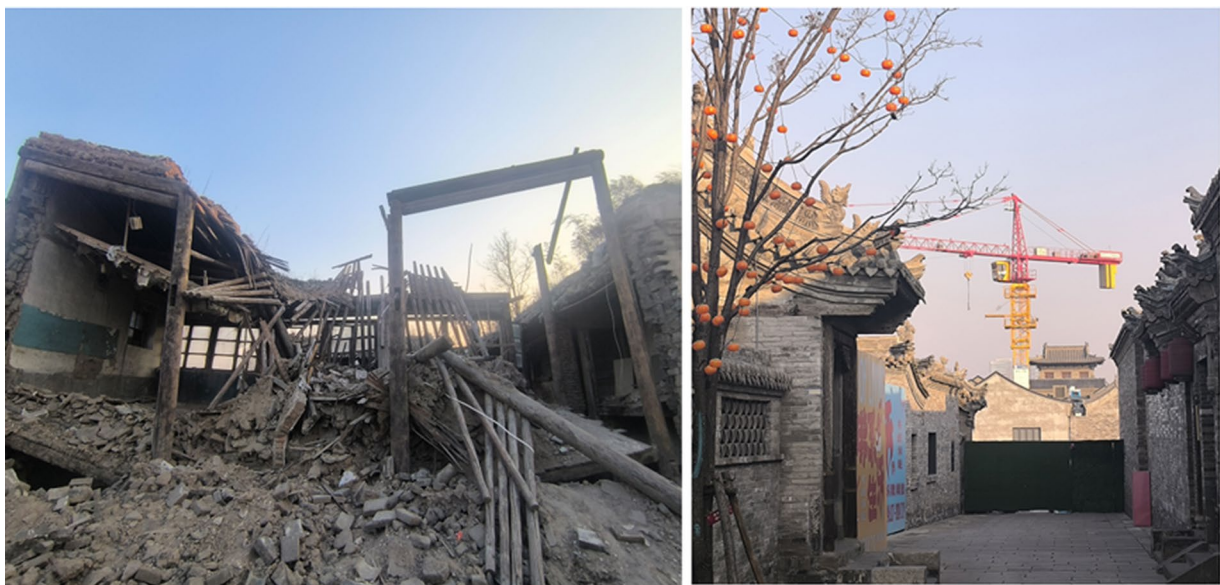
Figure 4. Datong Ancient City still under construction (Source: Author's photo, 2025).
