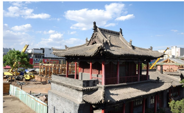
Huayan Temple under construction (2010)
