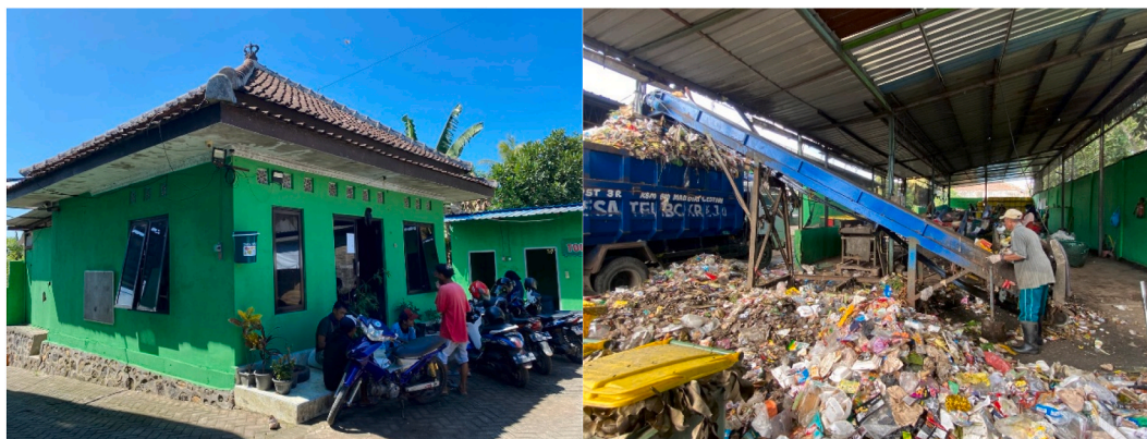
Fig. 2. Zero waste-based plastic waste pollution control facility.
