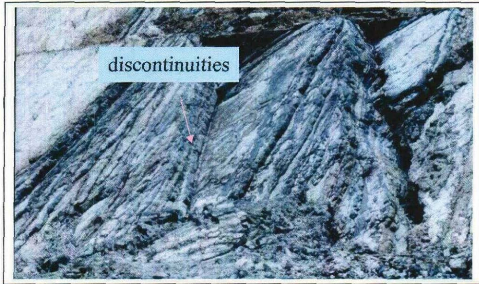
Figure 2.1: The discontinuities at CH 76000 of East Coast Expressway (2002)
