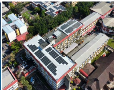
Fakulti Sains (528 kWp)
