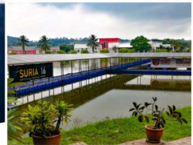
Floating Solar and Walkway (305.20 kWp)
