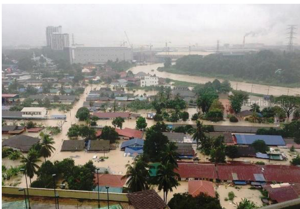
(c) The worst flood in Klang Valley on 19 Disember 2021
