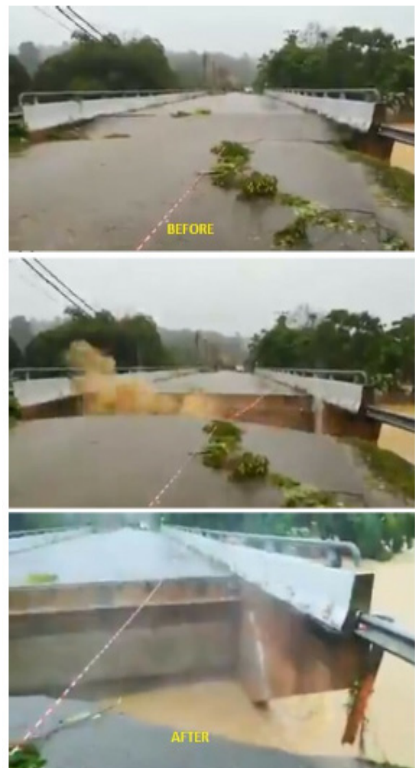
FIGURE 6. Bridge collapse in Raub, Pahang in January 2021 due to high discharge of river and extensive scour around pier and abutment.
