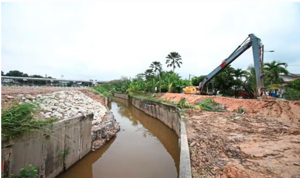
a) The Kg Melayu Subang flood mitigation project is scheduled for 2023.
