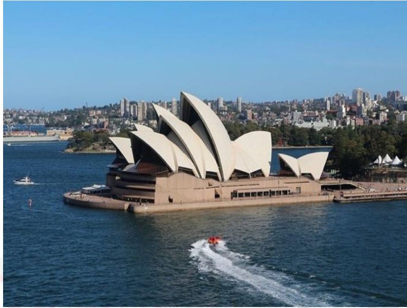
Figure 1.4: Sydney Opera House (Source: Bernard Gagnon, 2015)
