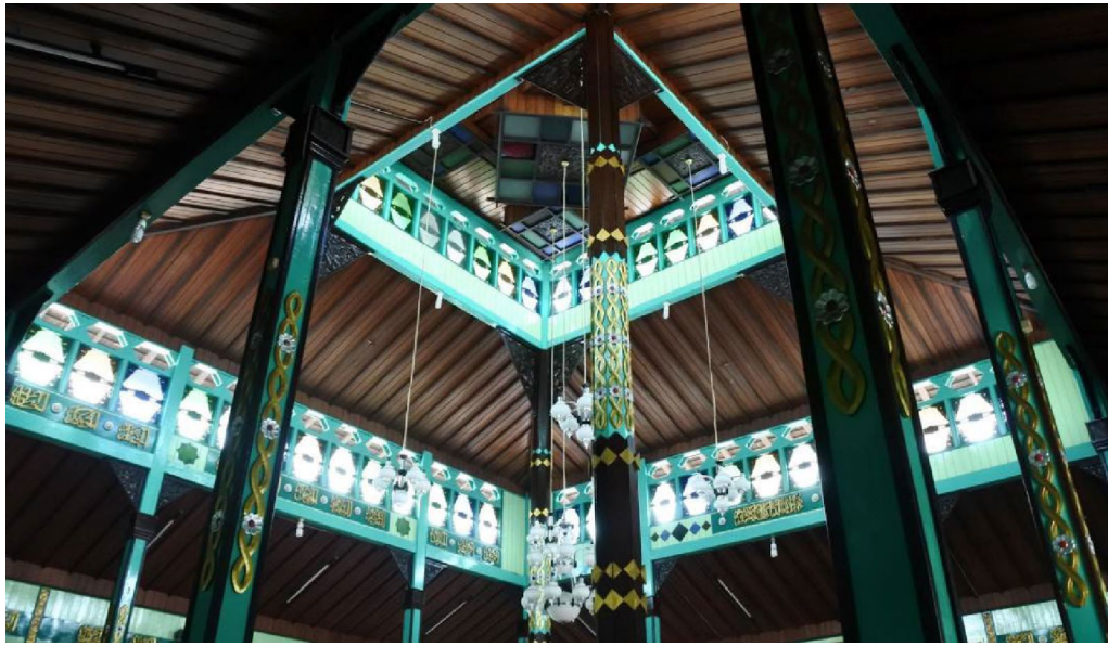
Fig. 16 Dome of the Sultan Suriansyah Mosque
