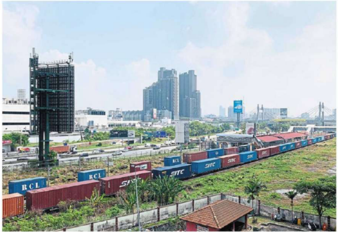
Railway overhaul: A file photo of KTMB cargo containers parked on tracks near the Setia Jaya station in Petaling Jaya. Experts say rail freight infrastructure needs to be improved to support the government's plan to shift more people and cargo away from roads under 13MP.
